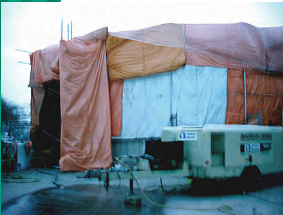
Vernon, BC. Digester Insulated Tarping Due to December Execution.
