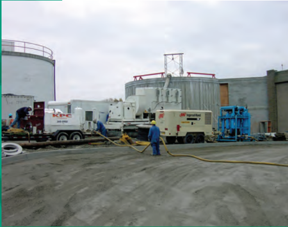
Vernon, BC. CCS Site Set Up.
