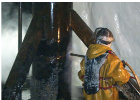
Stripping of Dock Ramp Column
