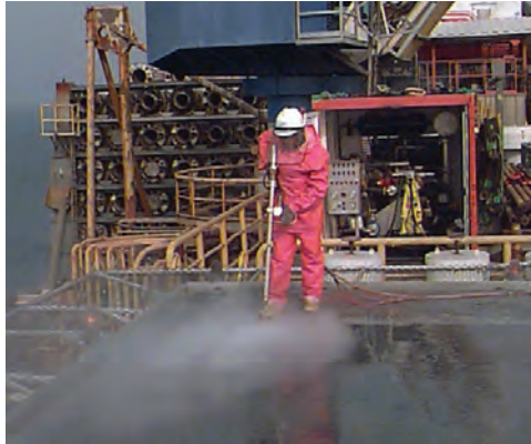
Surface Preparation of Heli-Deck on offshore Oil Rig
