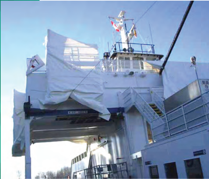
BCF C Class Ferry, Lead Abatement executed with UHP WJ
