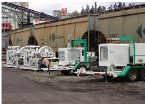
CCS Ultra High Pressure Water Jetting Fleet of Six Guns
