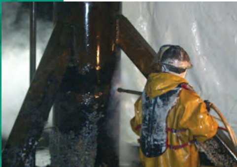
UHPWJ (40K) is not blast media reliant, generally lowering containment and waste management costs.
